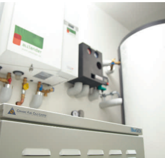
BlueGen-Anlage von Ceramic Fuel Cells.
